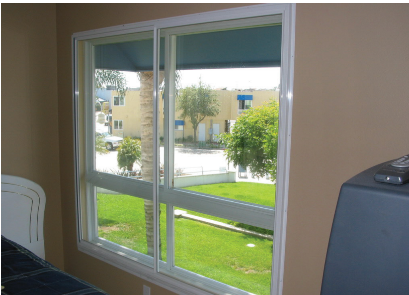
Guestroom with a second, inner soundproofing window
