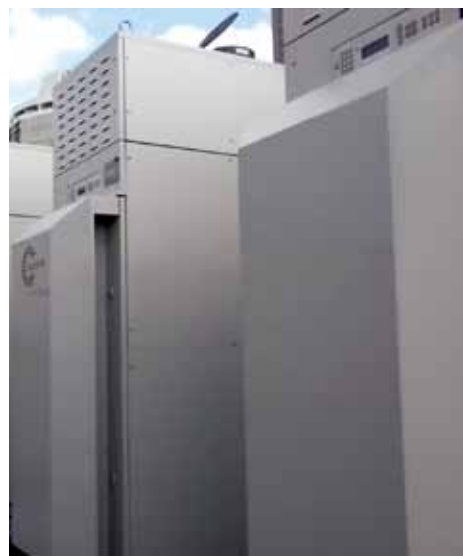
Three natural gas microturbines provide electrical and thermal power at the Four Seasons Hotel Philadelphia.
