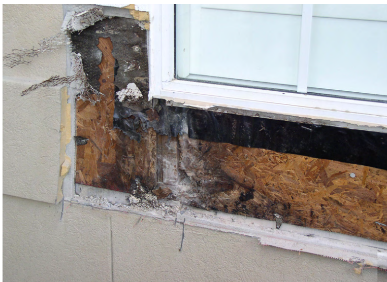
Multiple interfaces and components all exhibiting different thermal and dynamic movement create stress to the assembly.
