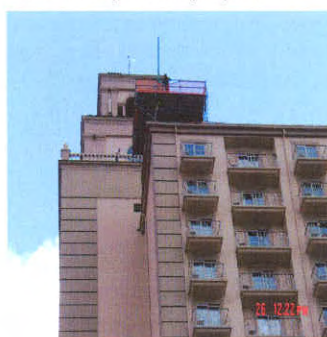
Roof top hydraulic hoisting stage area.
