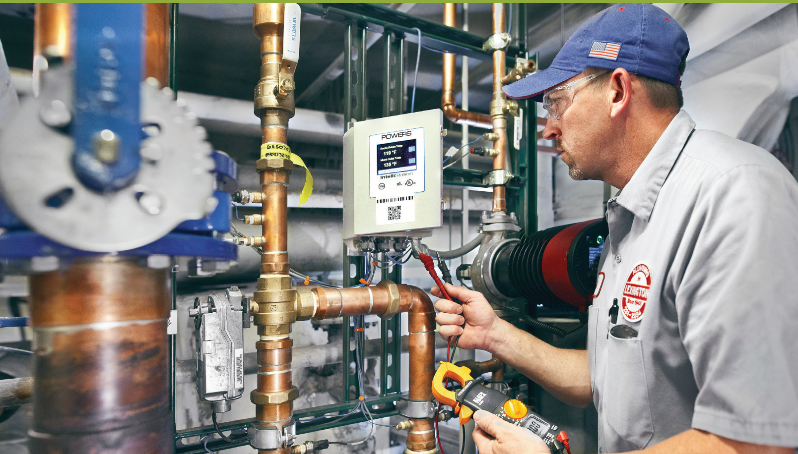
Joel Ryun, journeyman plumber, Lexington Plumbing, measures amp draw at the main control.
