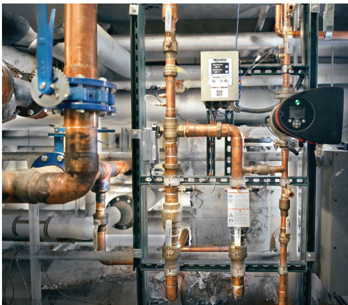
The IntelliStation digital mixing system at the Kansas City Airport Marriott hotel.
