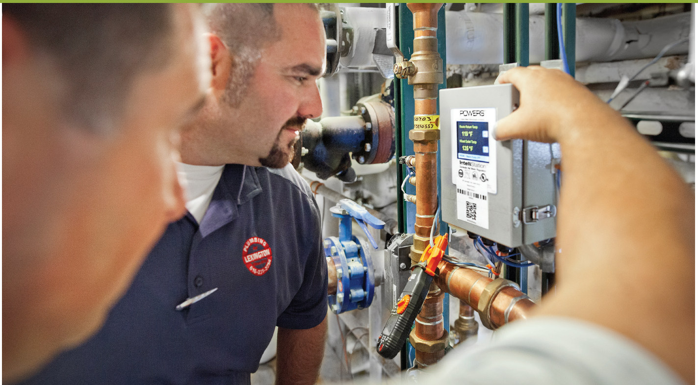
After making adjustments to the mixing valve, Ian Walters, project manager, Lexington Plumbing (center) and Jamey Shibel, outside sales for the manufacturer's rep firm, Mack McClain and Associates, determine the domestic water temperature setpoint.
