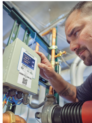
Ian Walters, project manager, Lexington Plumbing, sets IntelliStation setpoint and return temperatures.
