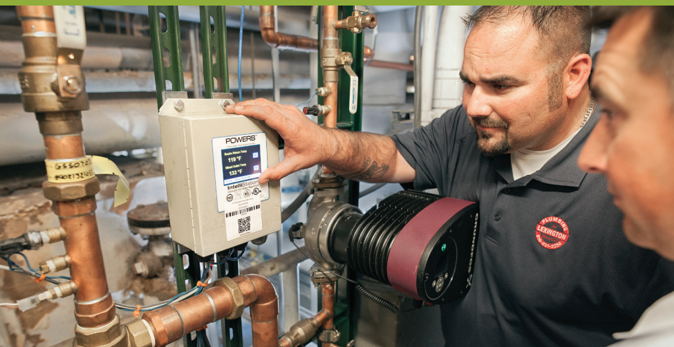
Ian Walters, project manager, Lexington Plumbing (left), and Jamie Shibel, outside sales for the manufacturer's rep firm, Mack McClain and Associates, make adjustments to the mixing valve's setpoint.
